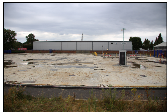
Current internal condition of site
